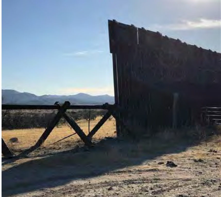
Approximately thirty minutes outside of Nogales, Arizona, the border wall transforms into "Normandy" barricades for several miles. Courtesy: Loyola University Chicago School of Law Immigration Law Practicum
